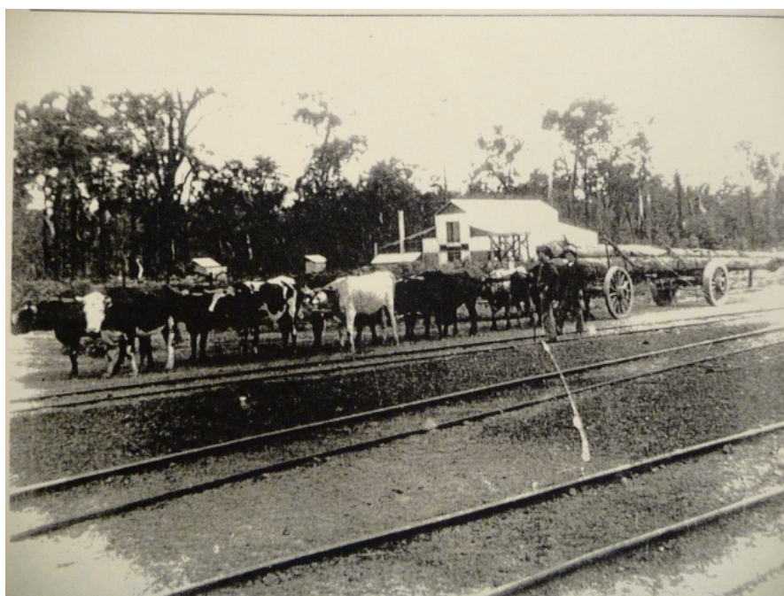
Photo 15 Bullock team with load of piles at Donnybrook Railway Station yard, with jam factory in background, c. 1918
