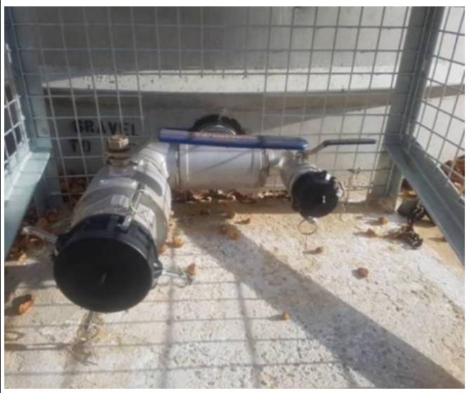
Strategic 47,000 Litre Concrete Tank & Protected Fittings
