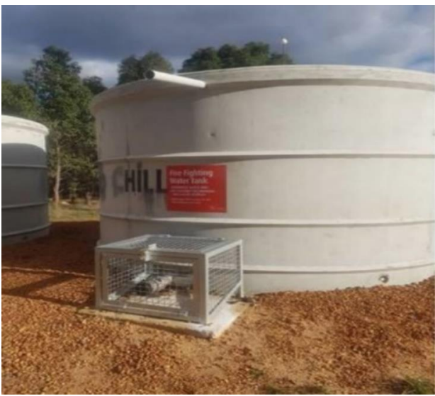
Strategic 47,000 Litre Concrete Tank & Protected Fittings
