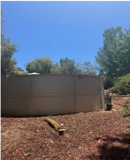
110 000L Rainwater Tank
